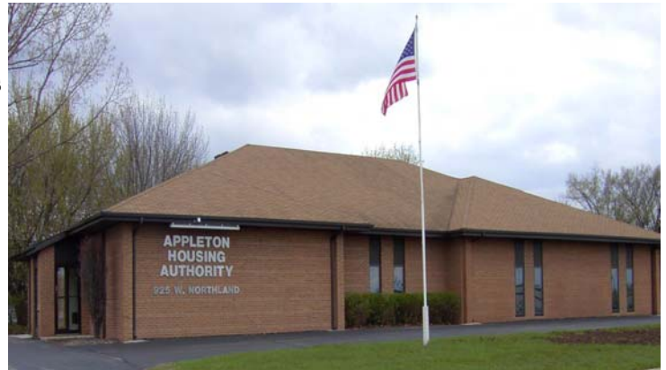
Appleton Housing Authority Main Office
